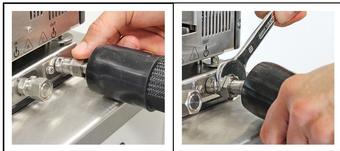
3. Screw the hoses onto the pump connectors by hand.
